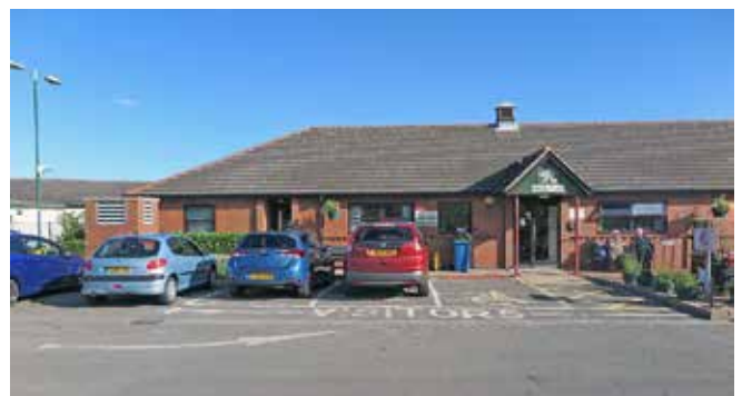
Rushcliffe Emergency Centre with tell-tale ventilation shaft on the left. Photo Clive Penfold
